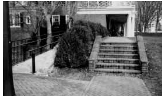
Modern ramp built adjacent to original shrubbery and stairs
