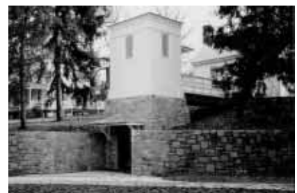
Elevator concealed in new outbuilding at Monroe Hill House
